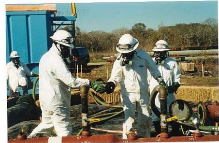
Custom design pigs and scrapers were developed to clean the pipeline.
