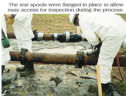
Test loop designed for evaluation of different thick film coating material for application to heavily pitted pipeline.
